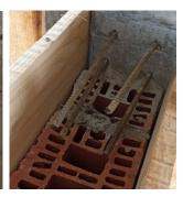
Figure 2. Execution of frame infill: a) classic masonry; b) anchoring; c) with horizontal cerclage. Case studies from Banja Luka, Bosnia and Herzegovina. Photography by authors, 2024.
