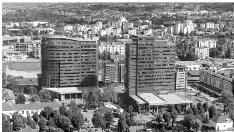
Figure 21. Urban Core 6 group form RS Government, office building and RTRS (Source: ekonferencije.com)
