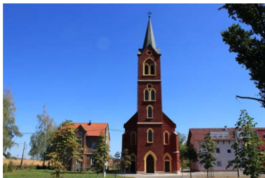
Figure 17 Convent of Holy family: parish house, church and new convent building; present condition [20]
