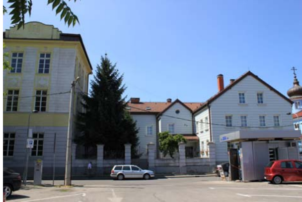
Figure 9 Convent of Sisters of Mercy of Saint Vincent De Paul. View of the Gymnasium and convent facilities; present condition [20]
