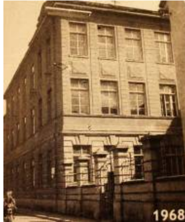
Figure 10 Catholic convent of Sisters of Mercy of Saint Vincent De Paul, Gymnasium in close-up view of main façade and courtyard side from north-west. Photograph taken 1968 [11:199]
