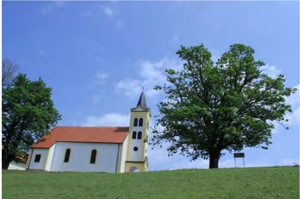
Church of Saint Michael the Archangel, Čelinovac: view from the west
