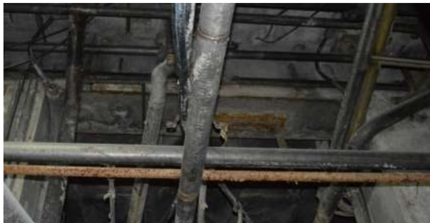
Figure 7. RC beam on which tests were carried out
