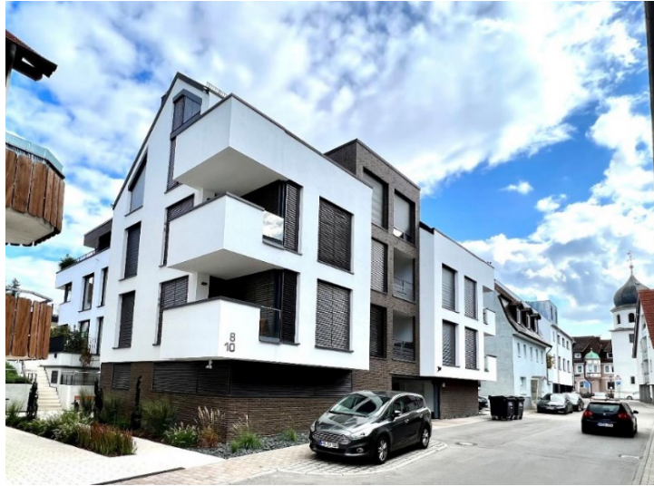
Figure 3: Street View along Offenauer Street with Old and New Structures [32]
