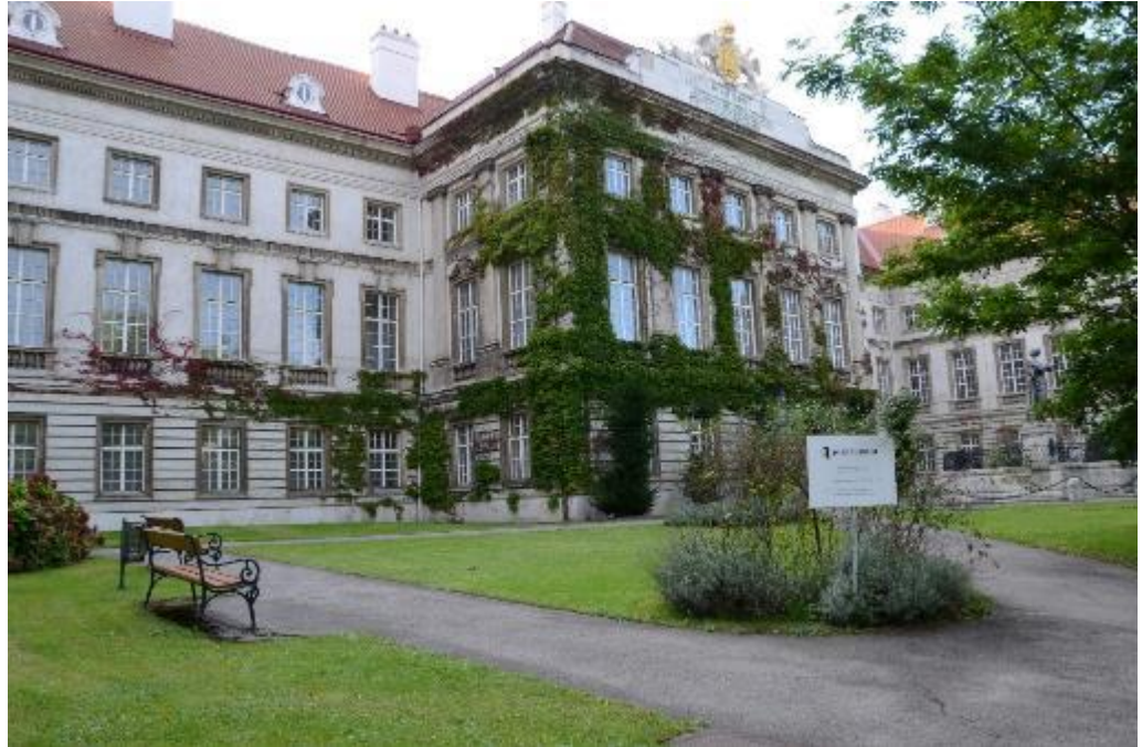
Fig. 4: The Josephinum building (1783-1785), designed by Isidore Canevale.
