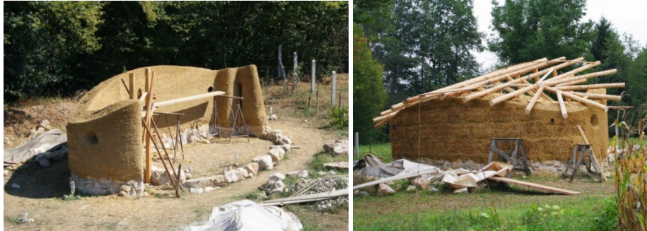
Figures 15. and 16. (Half)greenhouse, Banja Luka, Republic of Srpska, Bosnia and Herzegovina (2011-2014, arch. Ognjen Šukalo) during construction of the heat-retaining northern wall and roof structure. Materials: earth, straw, wood, glass. Photo: Ognjen Šukalo.
