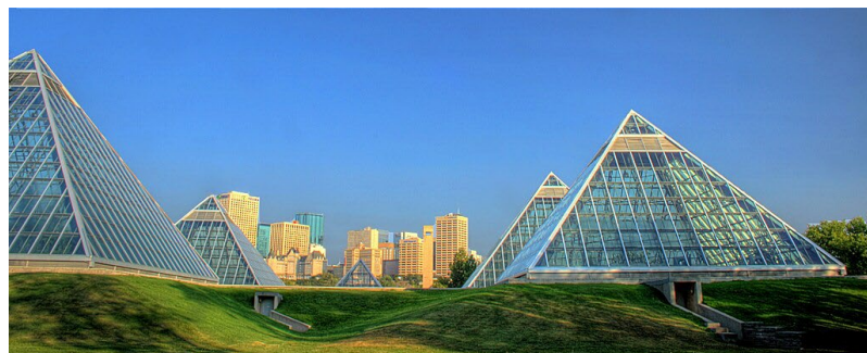
Figure 14: Muttart Conservatory in Edmonton, Alberta, Canada (1976, arch. Peter Hemingway). Excavated mounds provide both micro-climatic stabilisation and reduced energy use, as well as a finer relationship with the landscape. The translucent envelope efficiently shrinks into only four high points and almost minimal surface area. The ensemble significantly expands on entrenched notions of a greenhouse. Photo: WinterE229 Winterforce media, public domain.
