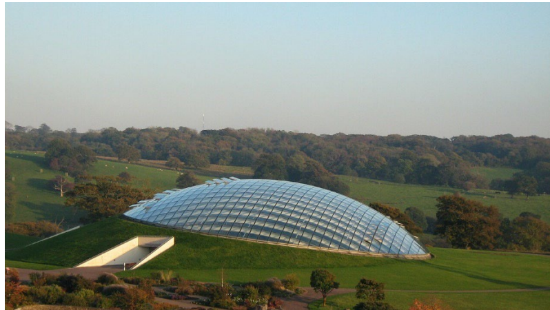
Figure 13: The Great Glasshouse at the National Botanic Garden of Wales (arch. Foster and Partners, 1995-2000). Besides being surrounded by embankment as a whole, the building has several additional indentations across the section in order to provide opportunities for heat capture and microclimate formation. Photo: Col Ford and Natasha de Vere, CC BY 2.0 Deed license.
