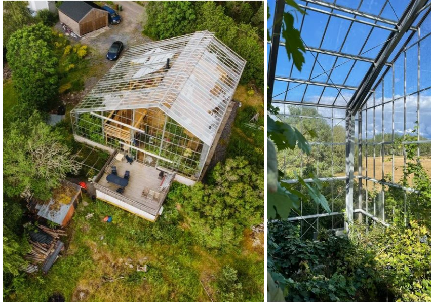
Figures 21. And 22.: Coupling and “hybridisation” of two types. The greenhouse dominates in the outer envelope but is, in turn, internally structured. Sundby Naturhus, Sweden (2014, Tailor Made Arkitekter). The Naturhus (natural house) concept of a house within a greenhouse was first extensively explored in the work of Swedish architect Bengt Warne in the 1960s and 1970s. Photo: Bjorn Wallentinus, Tailor Made Arkitekter and Greenhouse Living (general consultant).
