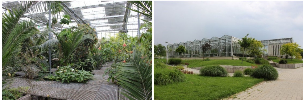
Figures 8. and 9. South Pest Wastewater treatment facility (Budapest, 2012, architecture: Organica Water, precise authorship unknown to us): Plants grown in a controlled environment assist in the process of aerobic/oxygenated fixed-film wastewater treatment.). Photo: Ognjen Šukalo
