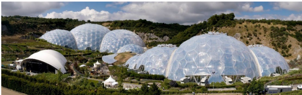
Figure 12: The Eden Project, Cornwall, UK (arch. Nicolas Grimshaw, 2001), the largest public/botanical greenhouse in the world. The envelope is comprised of a hexagonal-triangular tubular steel structure covered with inflated panels made of ETFE (ethyltetrafluoroethylene). Photo: Jürgen Matern, Creative Commons license BY-SA 2.5.
