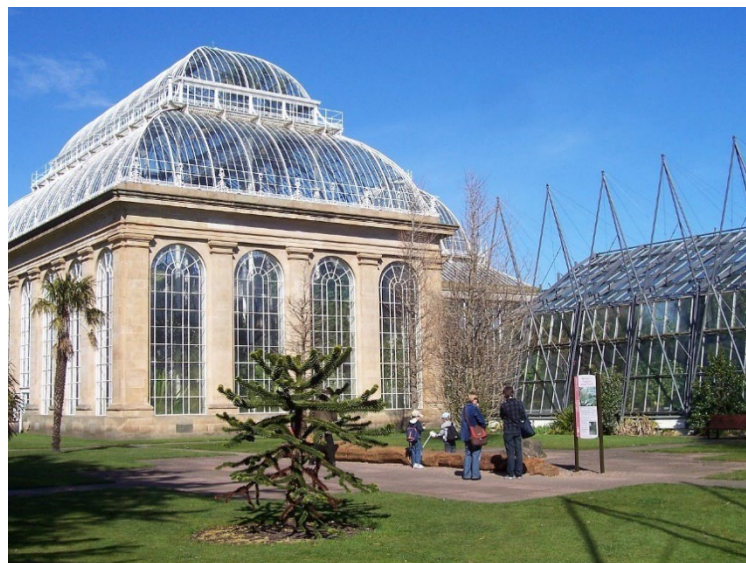
Figure 1. Glasshouses at the Royal Botanical Garden Edinburgh [4], displaying an array of periods and elements: on the left side is the Temperate Palm House (Matheson, 1858), with a substantial part of the solid-wall envelope (quite an unusual trait for the time, save for the orangeries of the previous era) and clearstorey central nave for the tallest of species. This building is also the highest XIX-century conservatory in Britain [4]. To the rear is the octagonal Tropical Palm House (unknown architect, 1834). The right side of the photograph reveals the Front Range (main glasshouse range, architects A. Pandreigh and G. Pearce, 1960) with its hi-tech structural exoskeleton. Photo: Andrew Bowden, CC BY-SA 2.0 Deed license.
