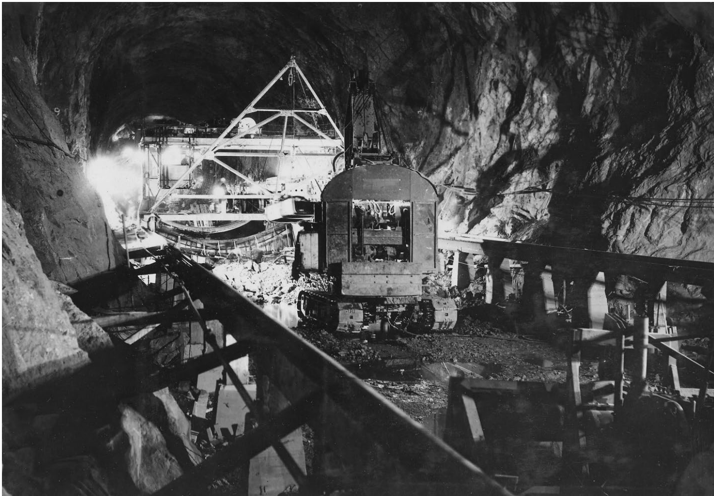
Photograph from Volume Two of a series of photo albums documenting the construction of Hoover Dam, Boulder City, Nevada, 1932. Source: National Archives and Records Administration, cataloged under the National Archives Identifier (NAID) 293677, Public domain, http://catalog.archives.gov/id/293677 (Wikimedia Commons)
