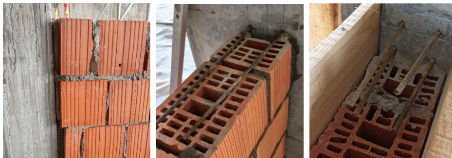
Figure 2. Execution of frame infill: a) classic masonry; b) anchoring; c) with horizontal cerclage. Case studies from Banja Luka, Bosnia and Herzegovina. Photography by authors, 2024.
