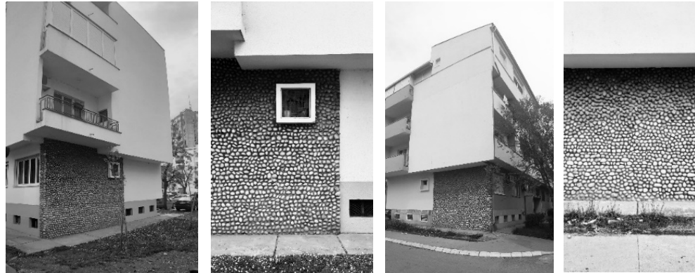
Figure 11. Residential buildings in Podgorica, 1960 and 1964 (photos by Danilo Bulatović)
